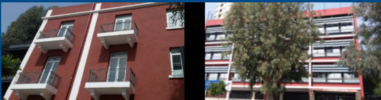
Figure 14: Examples of shading balconies and aluminum shading devices in Lebanon Source: Dr. Samir Traboulsi
