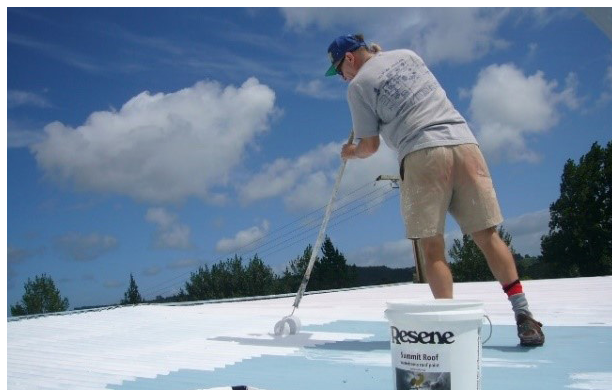
Figure 57: White roofs are on average 30 °C cooler than dark colored roofs in summer Source: White Roofs Project
