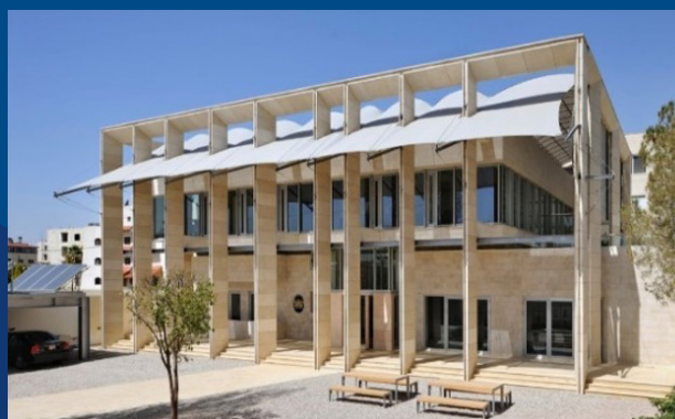
Figure 15: Shading measures on the Dutch Embassy Amman- Rudy Uytenhaak Architects Source: Pieter Kers
