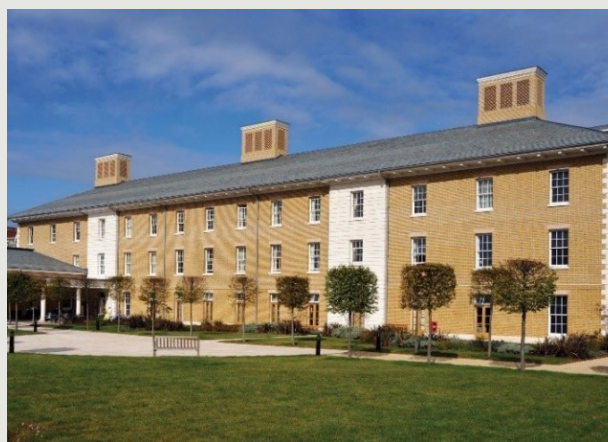
Figure 11: The Royal Chelsea Hospital in London, retrofitted with wind catchers for natural ventilation. Wind catchers originate from Middle East traditional architecture
