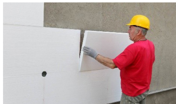
Figure 24: Outside polystyrene insulation Source: Milieucentraal
