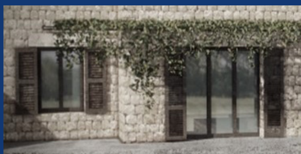
Figure 16: South facades and glazing-openings have been sheltered with horizontal overhang devices, sometimes with greeneries, allowing for ventilated/shaded buffers to be pleasant outdoor seating areas
