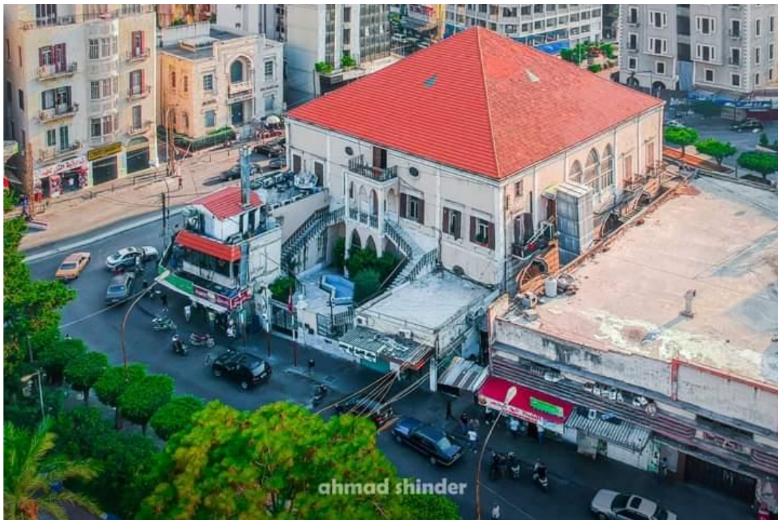
Figure 2 Drone picture of the Rashid Karami Municipal Cultural Center
