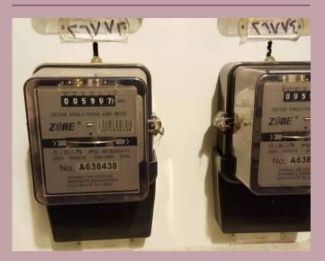
Net metering is a RE incentive through which consumers with small RE systems can offset the cost of power drawn from the utility. This works by installing a meter that records the bidirectional energy flow, allowing the excess power to be transmitted to the grid. The exported energy from the system is subtracted from the imported energy, and the net output is calculated. Net metering is a start-up tool used to promote clean energy through giving back incentives to customers.
