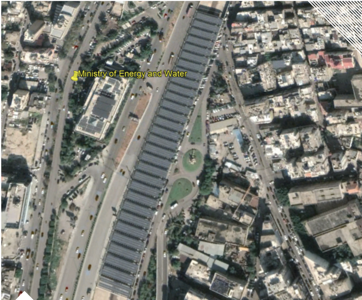
Figure 2. The one megawatt peak phase of the BRSS project. Adapted from Google Earth
